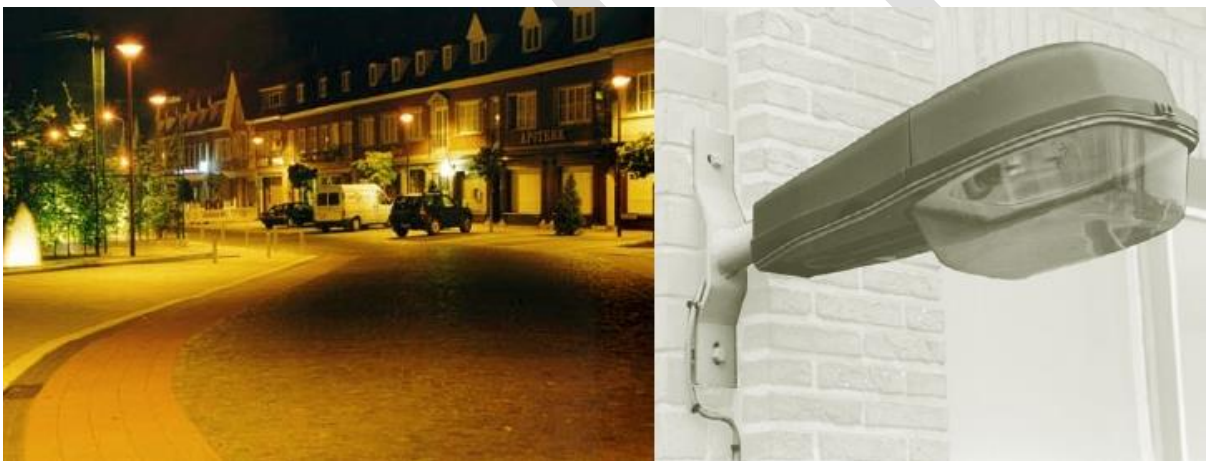
Figure 3-16: Street lighting luminaires attached to poles(left) and to a house (right)
