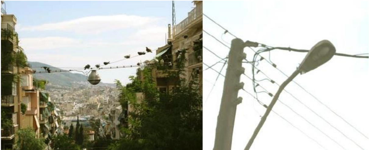
Figure 3-15: Street lighting luminaire attached to cables(left) and to electricity distribution (right)
